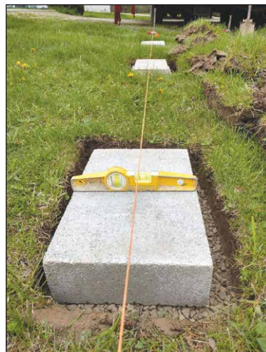
Individual block setting (shown above).
