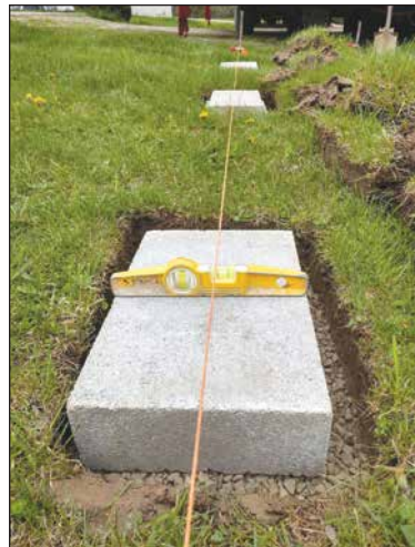
Individual block setting (shown above).
